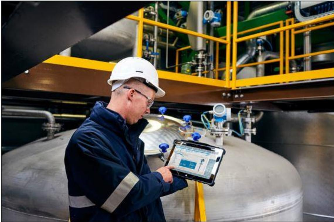
Endress+Hauser's robust, touch-enabled Field Xpert tablet PC (here: model SMT70 for Cl. 1 Div. 2) allows maintenance staff to manage virtually all digitally communicating E+H and other field instruments.
